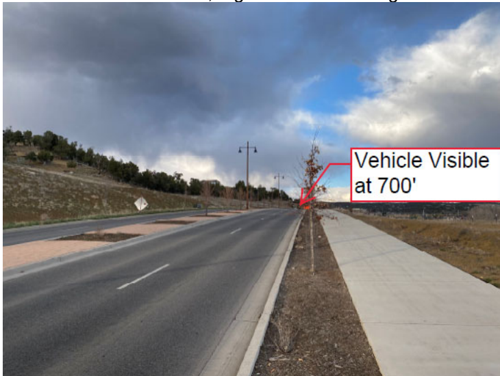
Exhibit 1 – East Entrance, Sight Distance looking East
